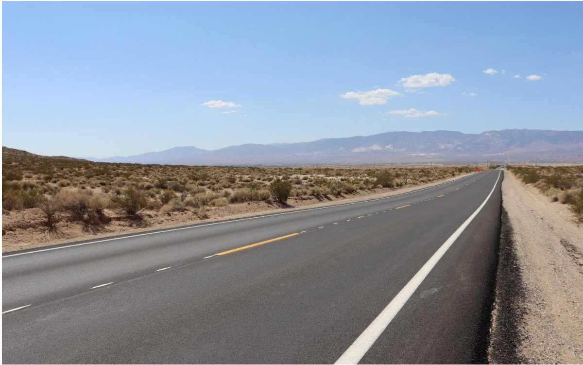
Photograph 1. Existing view looking southeast toward the Project area from SR 247 near Wilderness Road.
