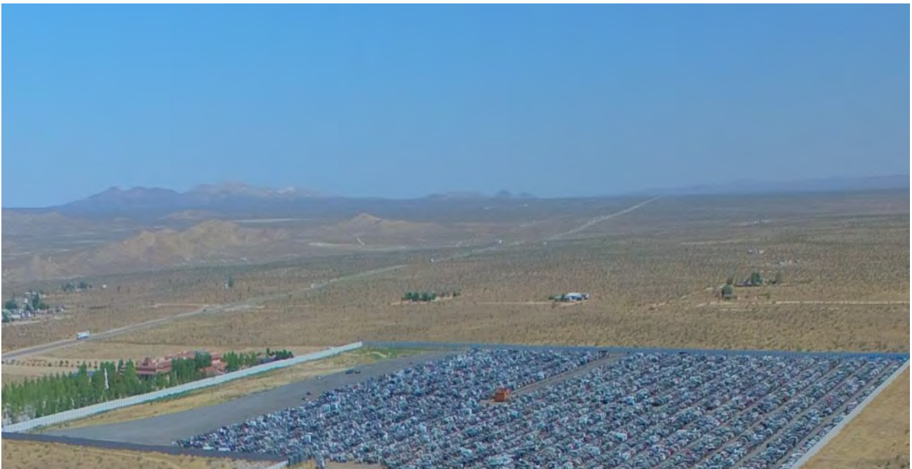
Photograph 2 - Looking North Across Site
