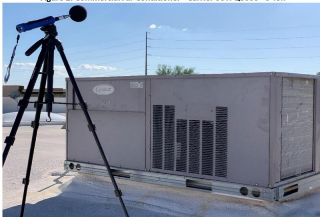
Figure 1: Commercial Air Conditioner - Carrier 50TFQ0006 - 5 Ton
