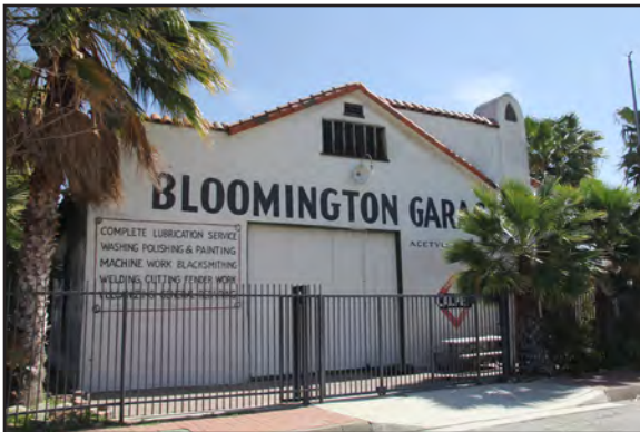
Historic Bloomington Garage at the corner of Commercial Street and Orchard Street.
