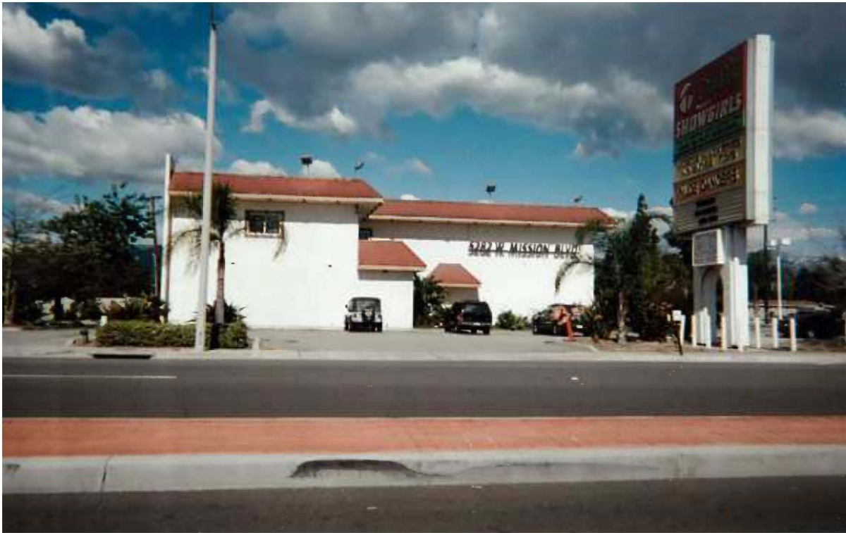
VIEW OF BUILDING FROM MISSION BLVD. (SOUTH SIDE)
