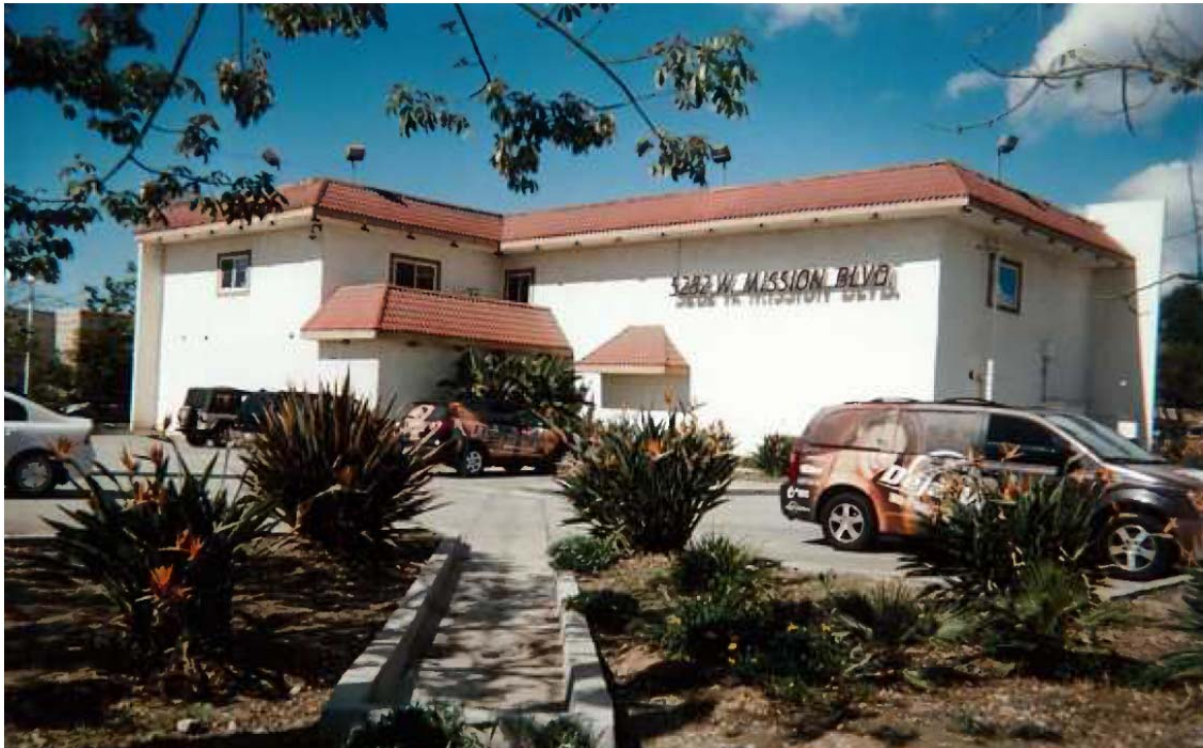
VIEW OF BUILDING FROM CORNER OF MISSION BLVD. AND CENTRAL AVE.
