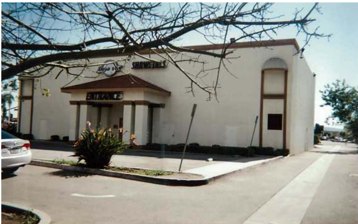
VIEW OF BUILDING FROM NORTH PARKING LOT
