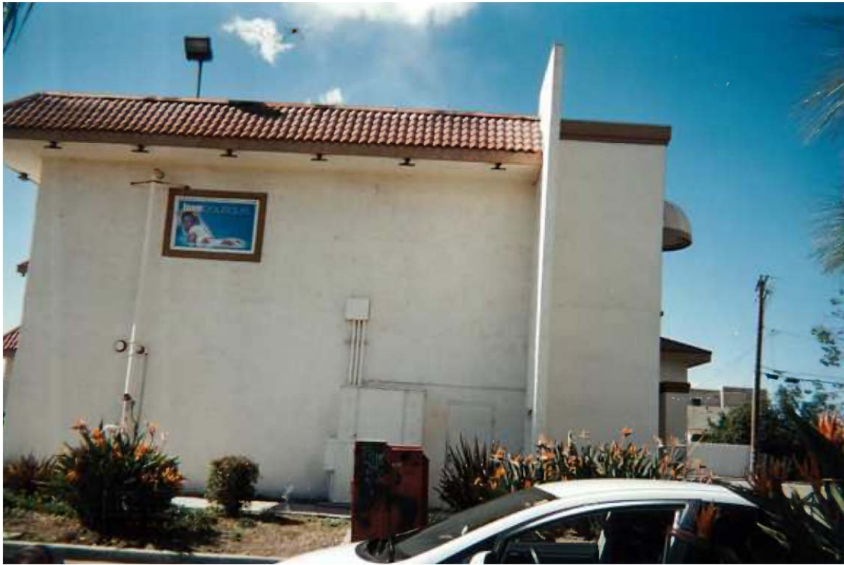
VIEW OF BUILDING CENTRAL AVENUE (EAST SIDE)
