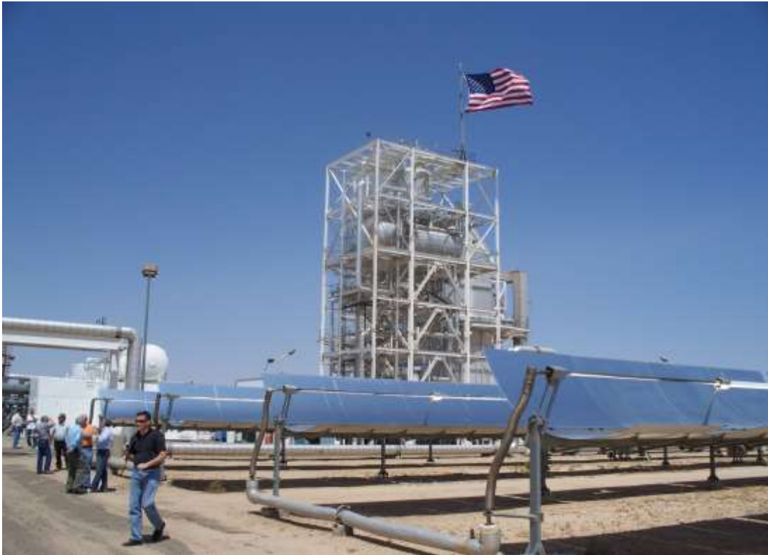
Existing field in the foreground with power block in background
