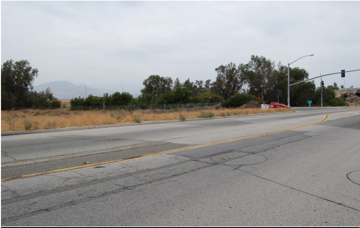
SAN BERNARDINO AVE. AT 210 FWY SOUTHBOUND OFF-RAMP
