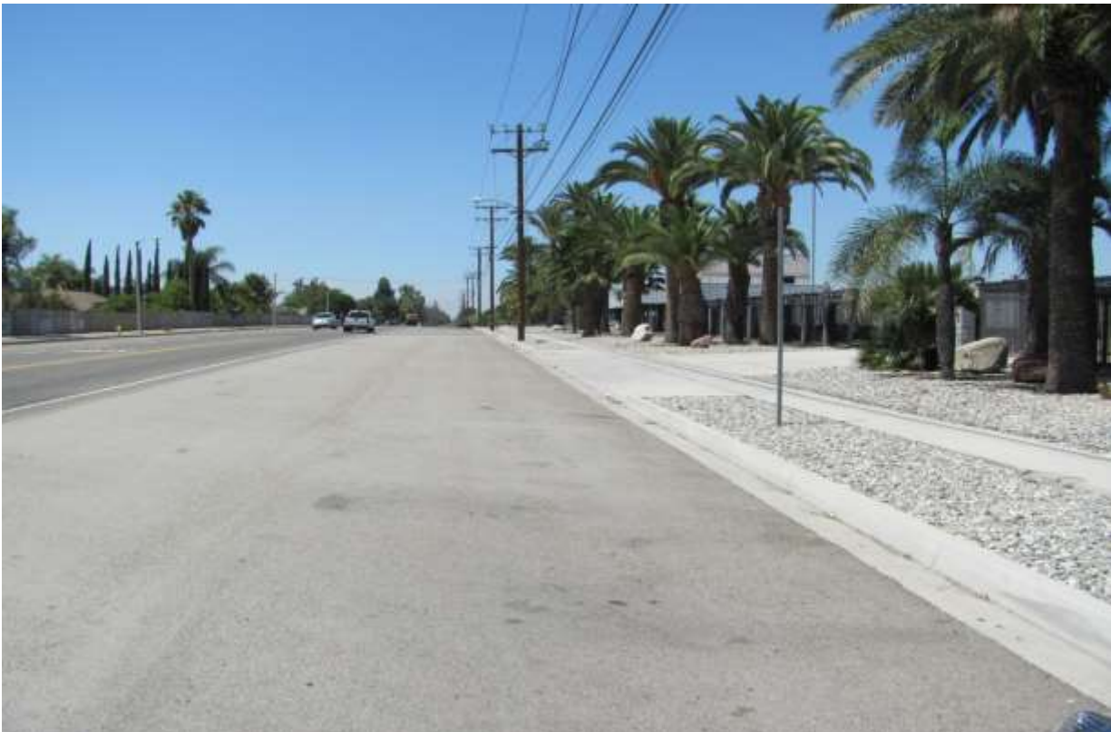
LOOKING WEST ON SLOVER AVENUE
