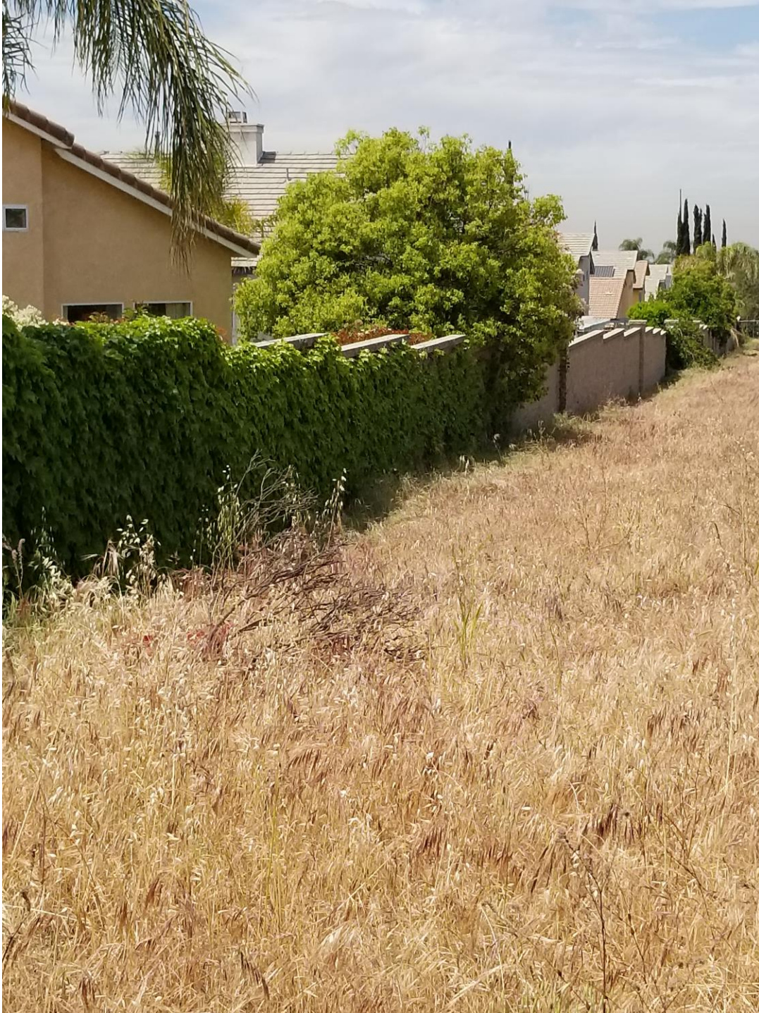
Figure 7: View of Existing Block Wall between the Property and Adjacent Subdivision
