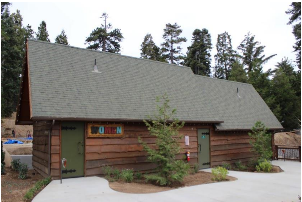
Existing Restroom Facilities
