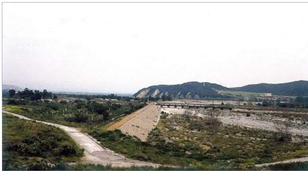
Flood control facilities within the site
