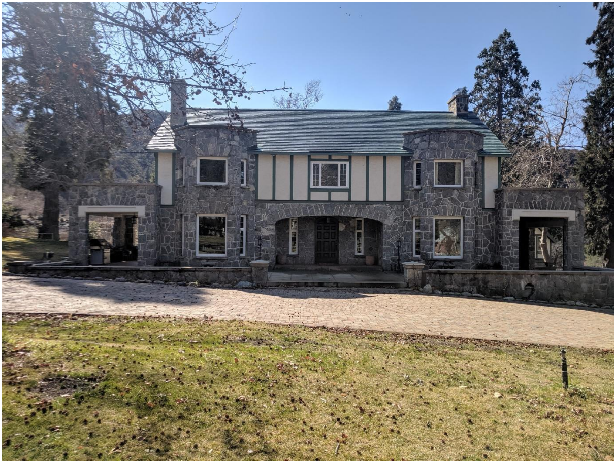
Figure 1 Front View of Home
