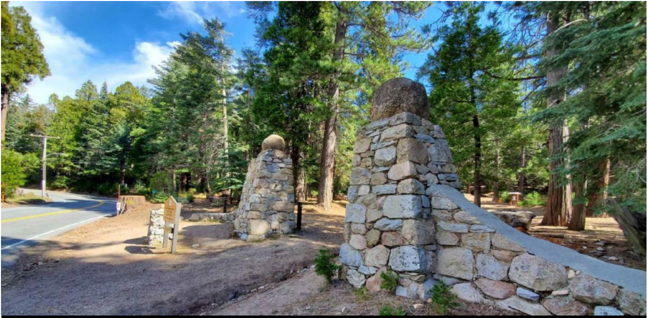
Figure 4 View of Site Entrance on Highway 189
