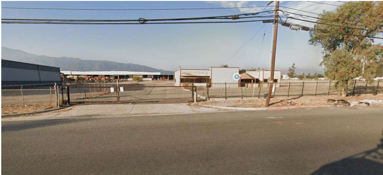
Looking north at the Project site from Arrow Route; the existing structure holding offices and fence to be demolished to allow for new construction
