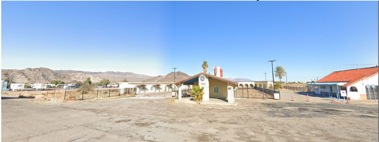
FIGURE 11 - Vacant Motel Facility
