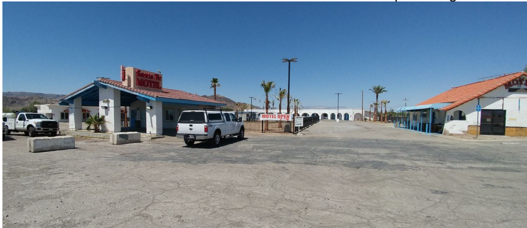
FIGURE 18 - Motel office and former office Gift Shop Buildings
