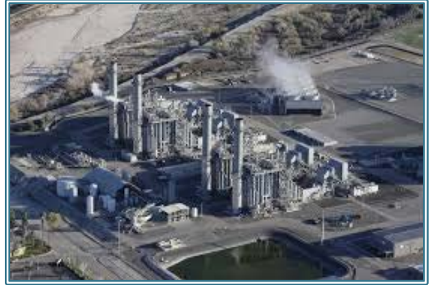
Southern California Edison's Mountainview Generating Station in San Bernardino County is the most polluting power plant is one of the largest contributors of greenhouse gas emissions in the state according to the Environment California Research & Policy Center.
