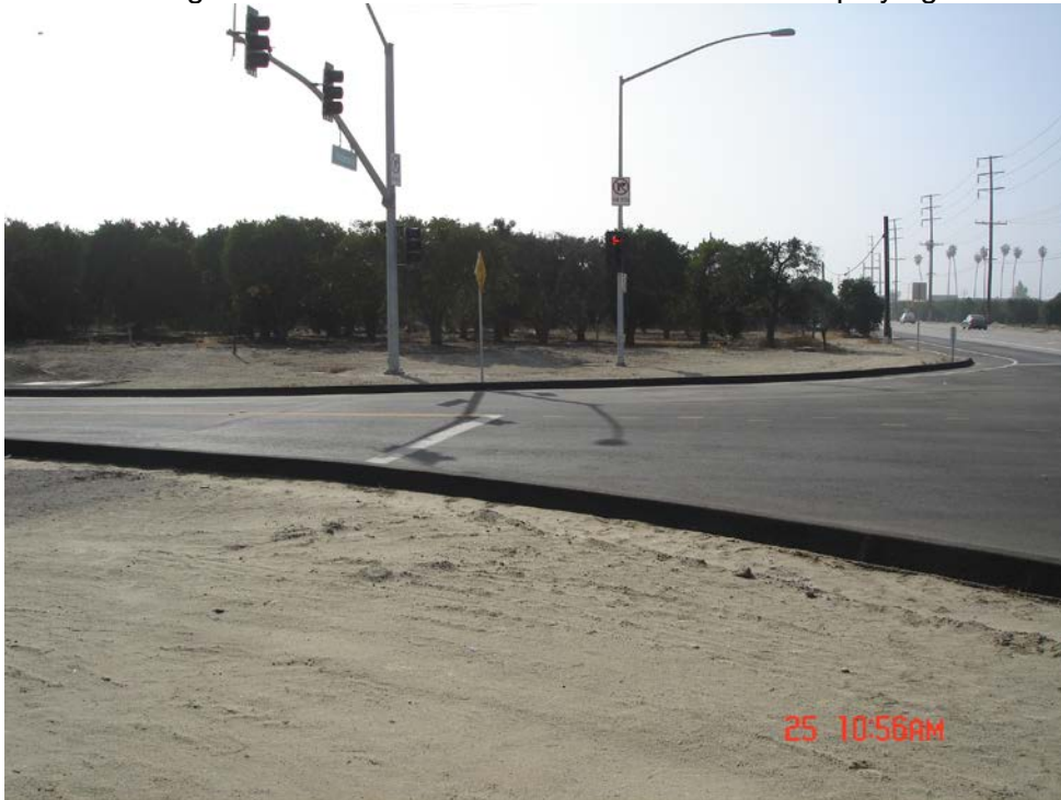
View to the South along Alabama Street at Palmetto Avenue and displaying new traffic signals.
