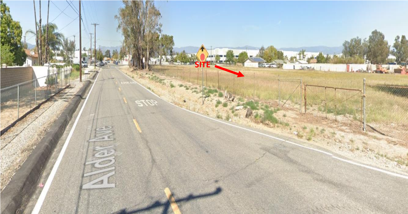
Photo 6 - View of site looking north from Alder Avenue
