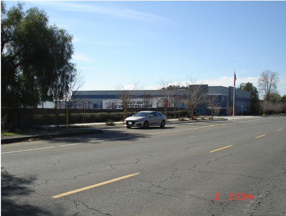
View westerly onto the adjoining property.
