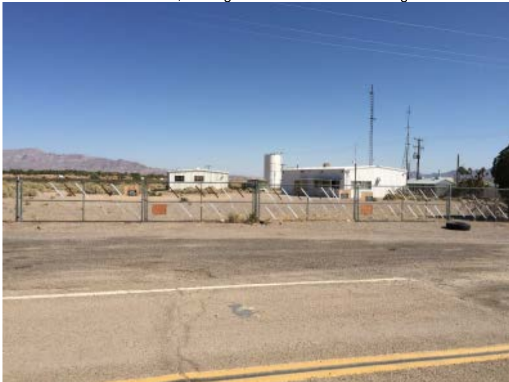
On Yates Well Road, looking north-northwest at buildings on site..
