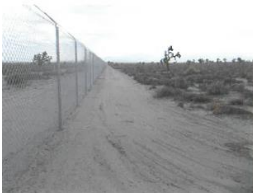
Figure 6 Northeast Corner of Property Looking South
