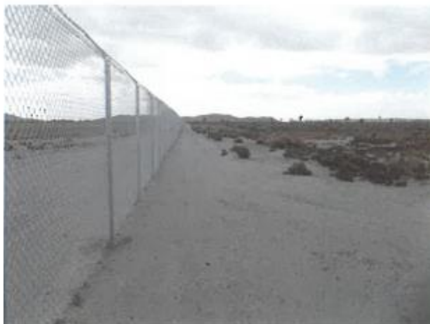
Figure 9 Southeast Corner of Property Looking West
