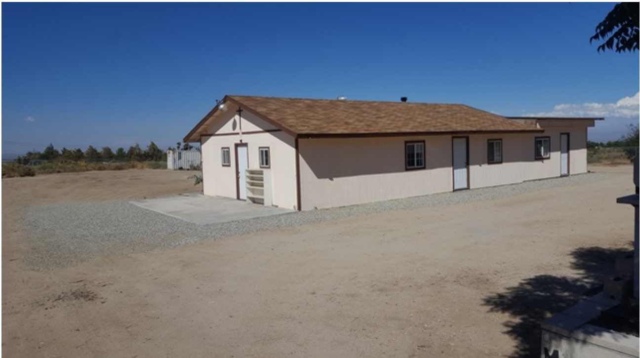
Metal building in rear of parcel.
