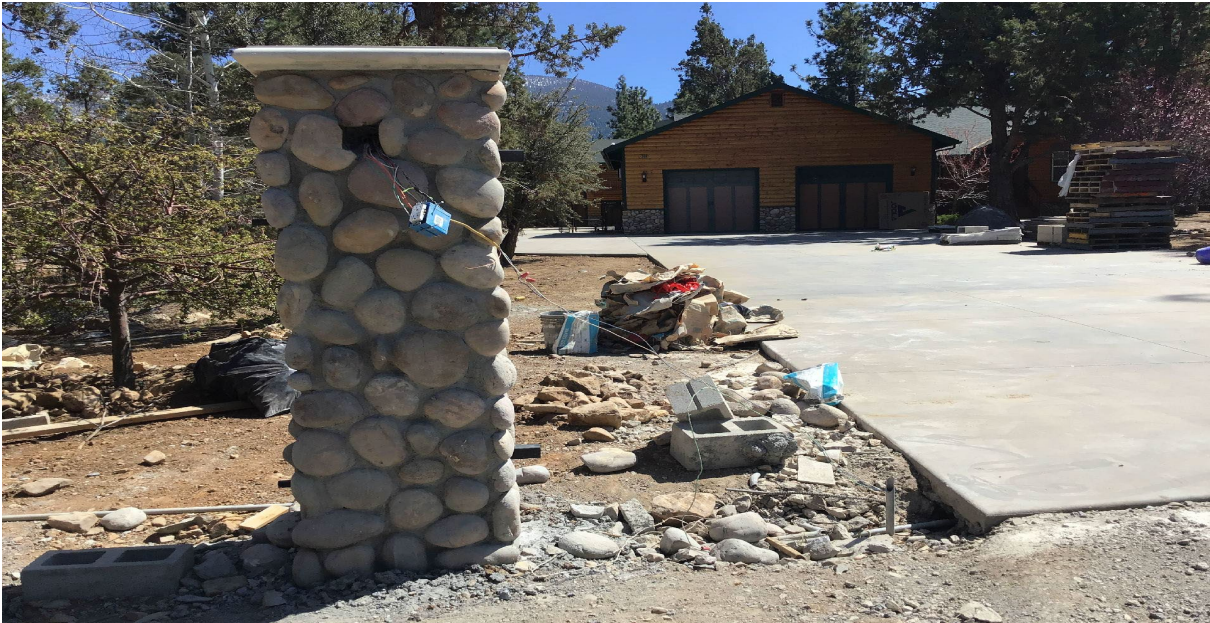
View of the 6-foot high block pilaster within front yard setback.
