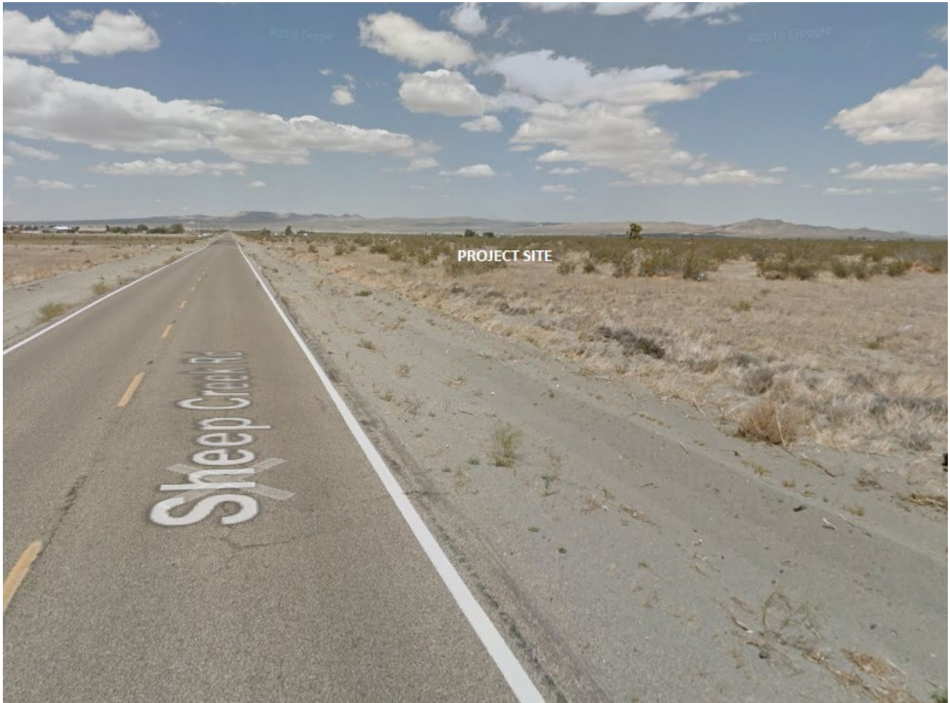
Figure 4 Sheep Creek Road looking north - Project site on right
