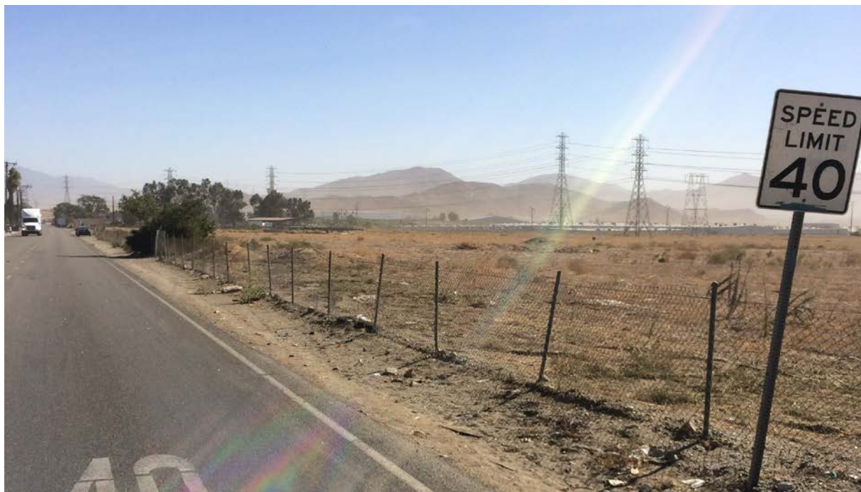
AT NORTHERN PROJECT BOUNDARY LOOKING EAST ALONG JURUPA ROAD
