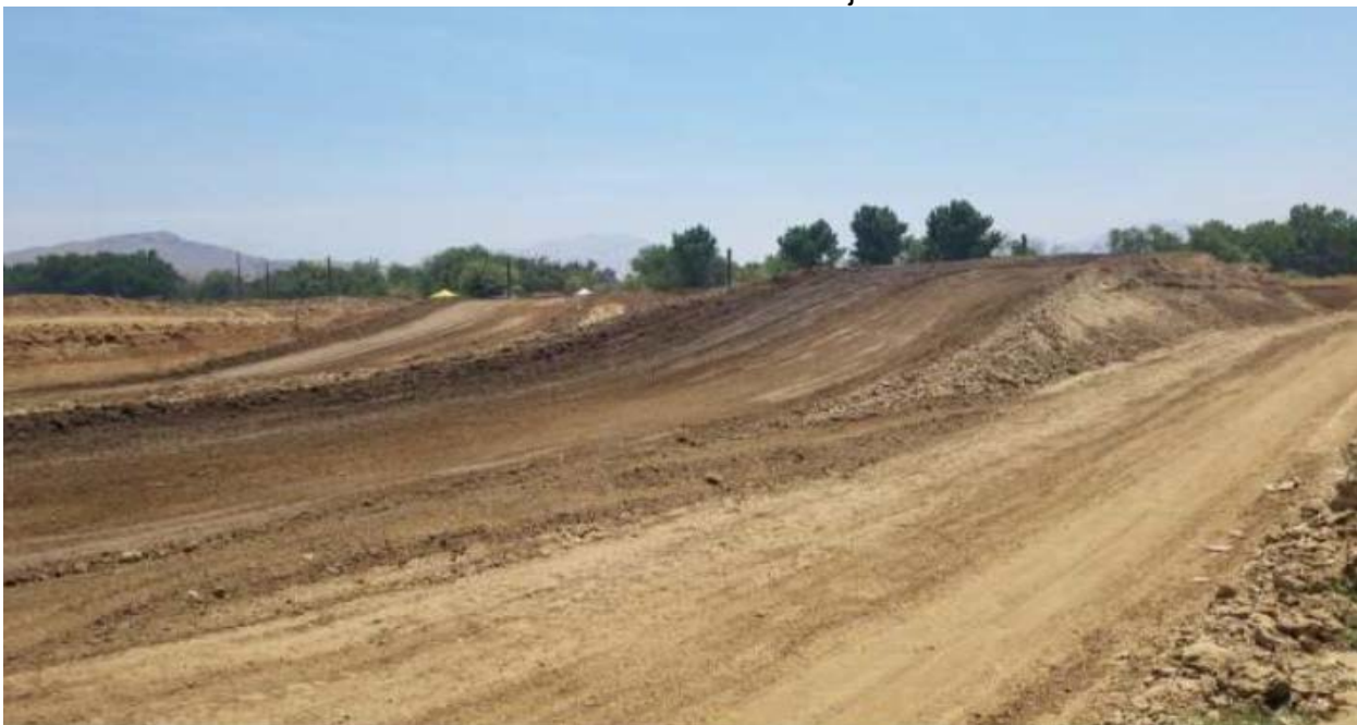
South view from the Project Site
