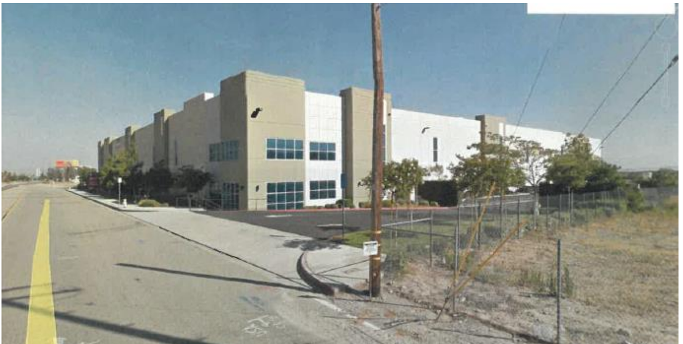
Northwest view from Kendall Avenue
