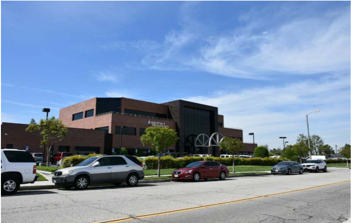
Looking south across Lugonia Ave.
