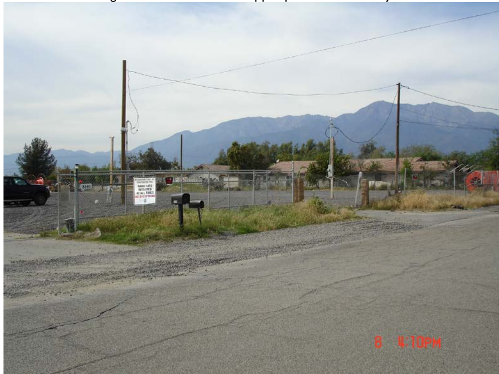
Looking northwest across the upper portion of the Project Site
