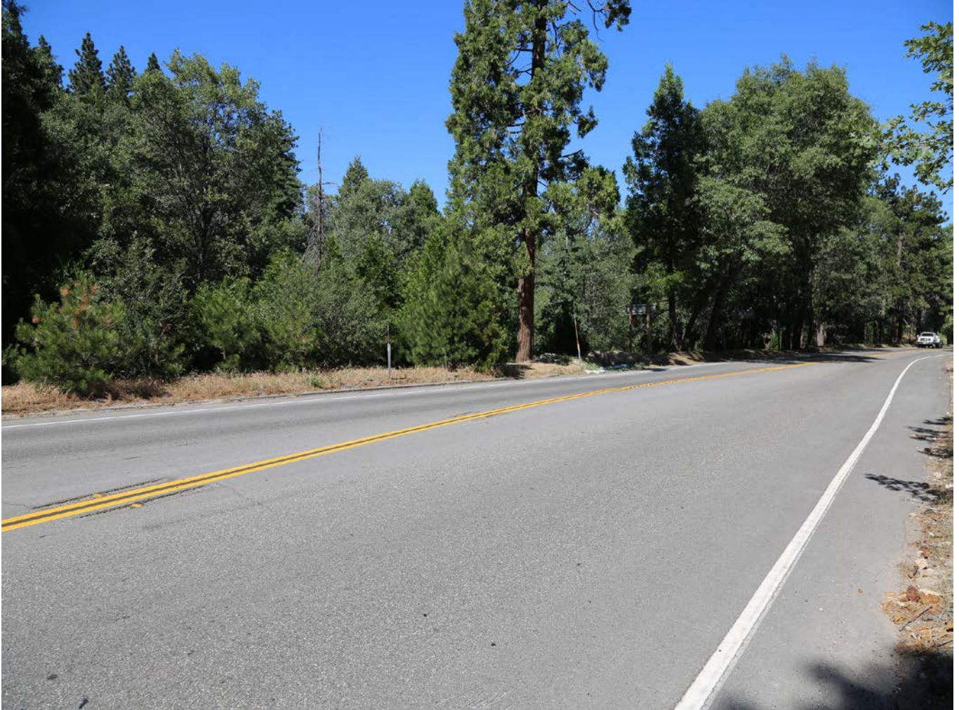
LOOKING NORTHEAST ALONG STATE ROUTE 18 AT WEST END OF PROJECT
