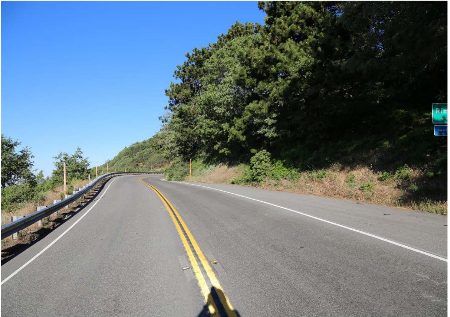
LOOKING WEST ALONG STATE ROUTE 18
