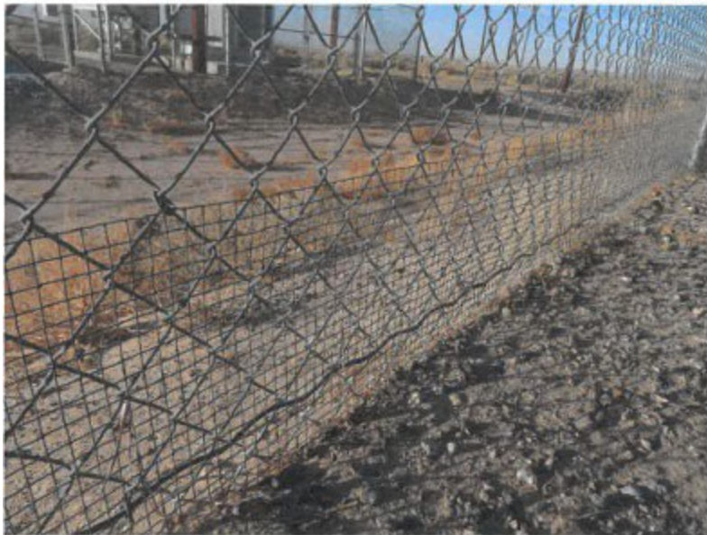
Figure 3 Existing Tortoise Fencing
