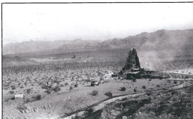
1934 photograph of the primary rock crusher with the narrow gauge tracks in the foreground leading from the quarry to the crusher. The buildings in the distance in the center of the photo were the secondary crusher and the kilns at the railroad. View is to the east. Old Woman Mountains in the background.
