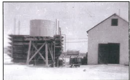
Undated photo showing details of the corrugated tin shed that housed the diesel generators at Chubbuck. The water tank and cooling tower used to cool the circulating water for the motors is on the left. An ore car sits on the narrow gauge track in the background.
