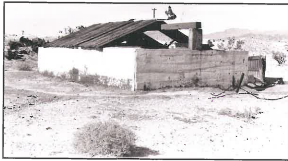
1977 photo of the oil bunker at Chubbuck used to store crude oil that was piped to the kiln burners. Although the roof is now gone, this is one of the few structures that still survives.
