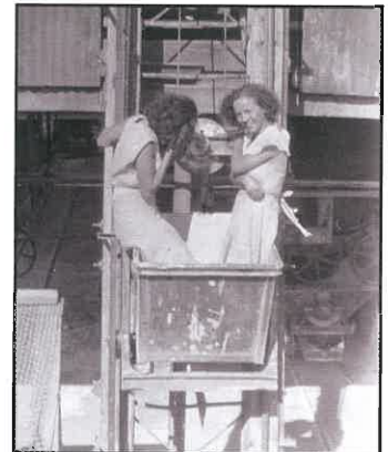
Bertha Piper (left) and Margarite Piper (right), playing in the ore bucket in 1932. When filled with crushed lime the bucket was hoisted to the top of the kiln via an inclined track visible in the center of the photo behind the girls' heads.
