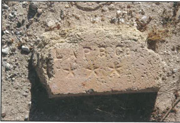
A discarded piece of fire brick from the vertical kilns lying on the ground at Chubbuck. The initials L.A.P.B.C. stand for Los Angeles Press Brick Company.
