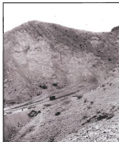
The limestone quarry at Chubbuck, 1934. Narrow gauge tracks were put down in several places for ore cars to be brought up to the rock face. Once loaded the cars were pushed to the primary crusher. The total amount of limestone taken from the mine is estimated to be 10 to 12 million tons.
