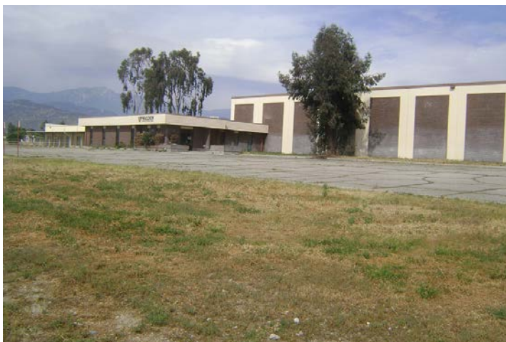
Front of main warehouse building from Opal Ave.
