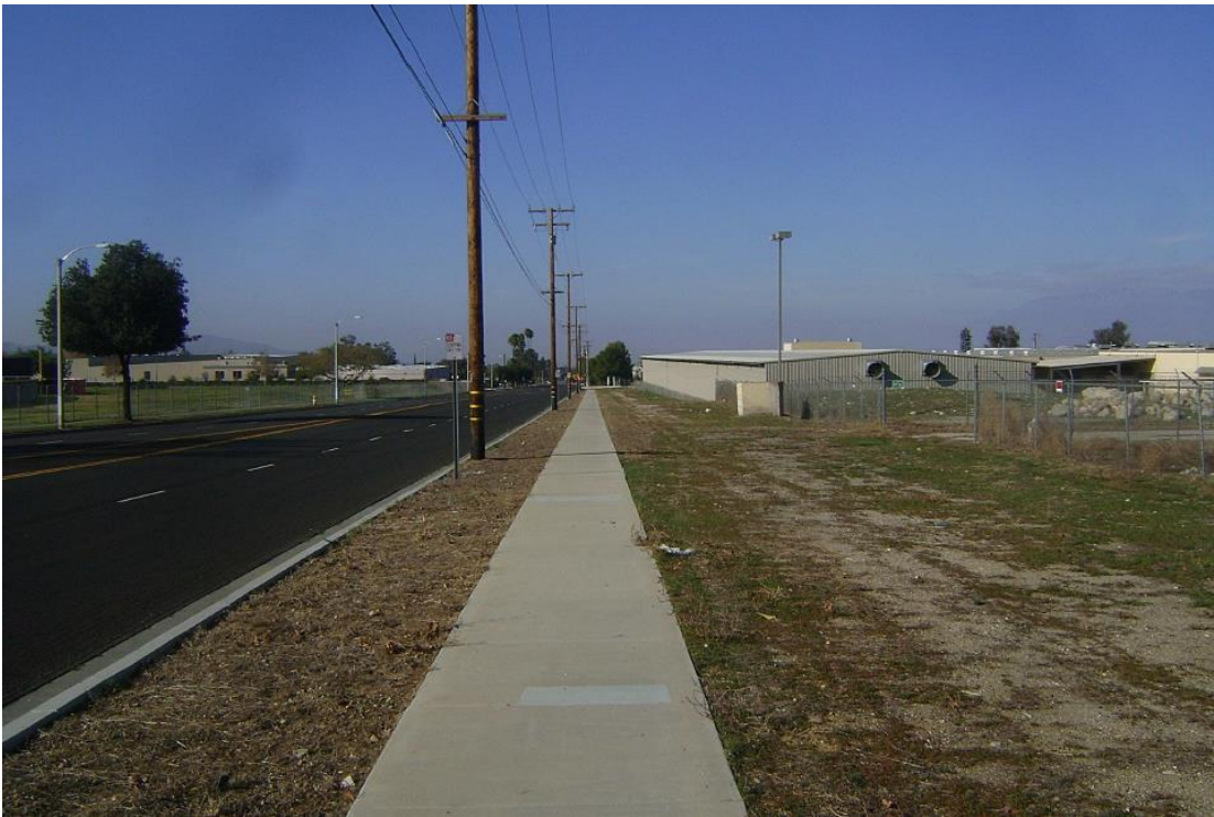
View along Colton Avenue looking west
