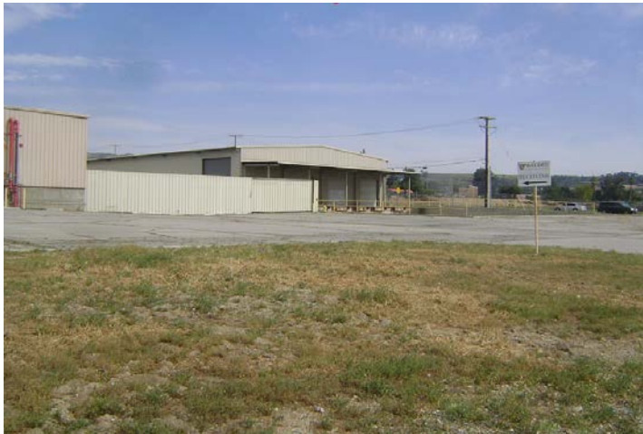
Front of small warehouse building from Opal Ave.
