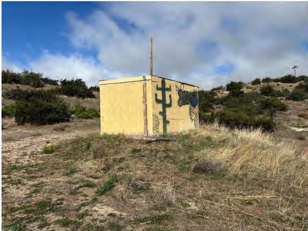
Project overview. View looking west at a well house
