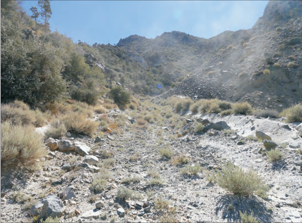
Photograph 11 - View of non-jurisdictional road cut. View to the southwest.
