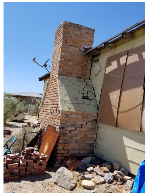
Figure 2: Chimney damaged in Trona Earthquake
