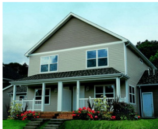
Duplex from Nogi Gardens Development Courtesy of California Manufactured Housing Institute (CMHI)
