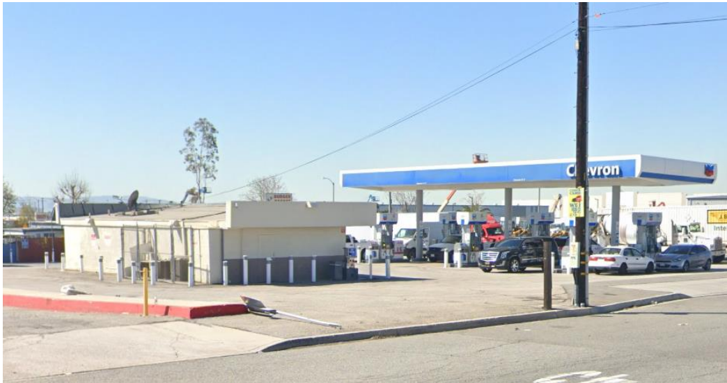
Figure 3: From the rear of the project site looking east.
