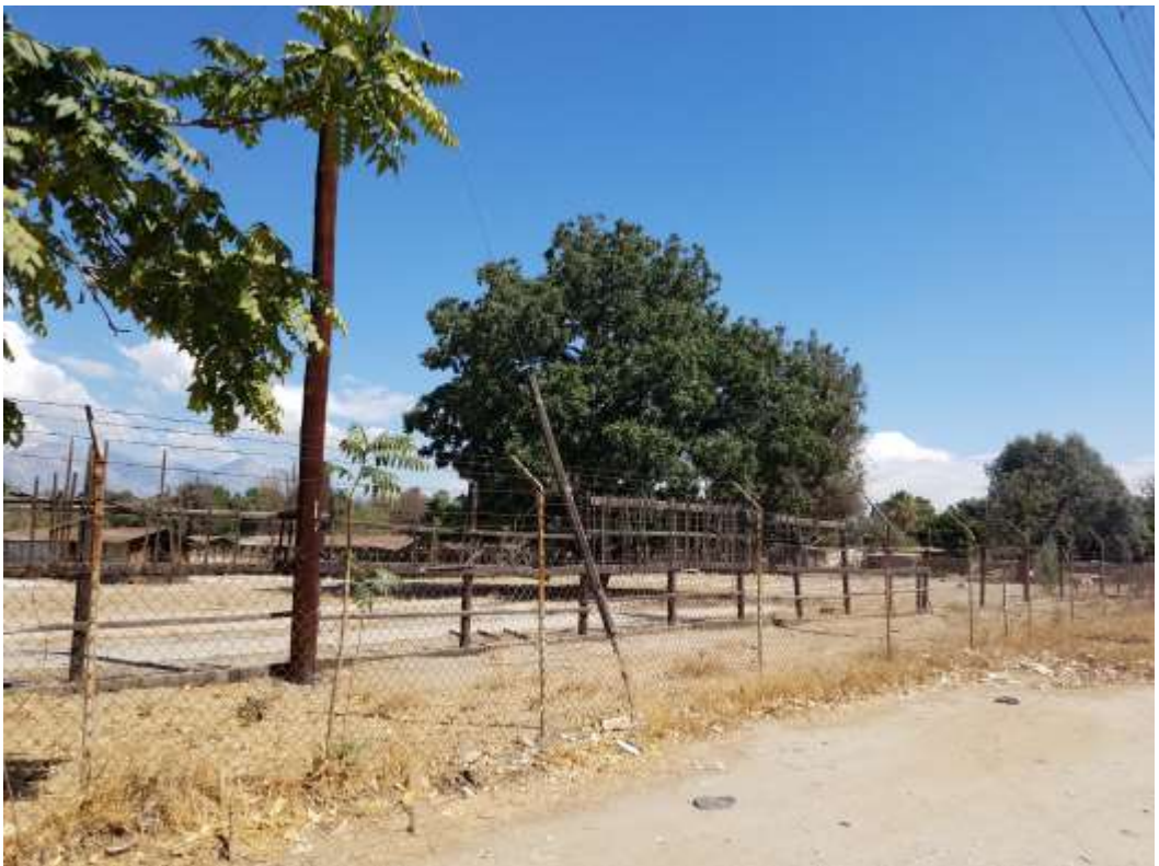
Figure 2. Yorba and Francis Property Fence and Structural Remains - View East
