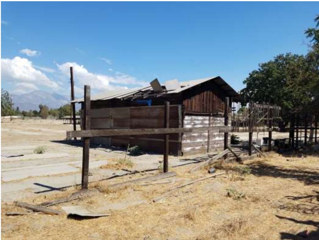
Figure 6. Yorba and Francis Outbuilding – View East
