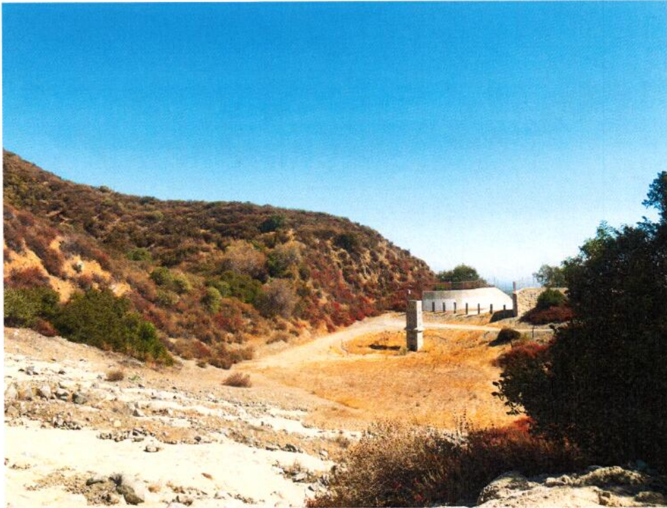
WEST SIDE OF SITE LOOKING SOUTH EAST
