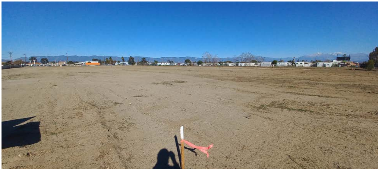
Photograph No. 1, Present site conditions facing northeast from the eastern edge of the infiltration basin.
