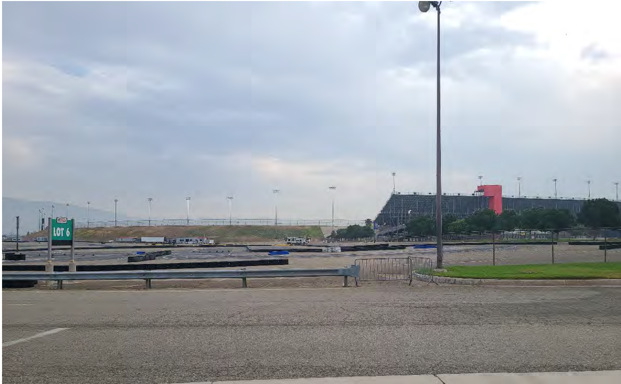
Figure 5-3. Overview of parking lot (foreground), raised outer bank of speedway (background, left) and stands (background, right), looking north.
