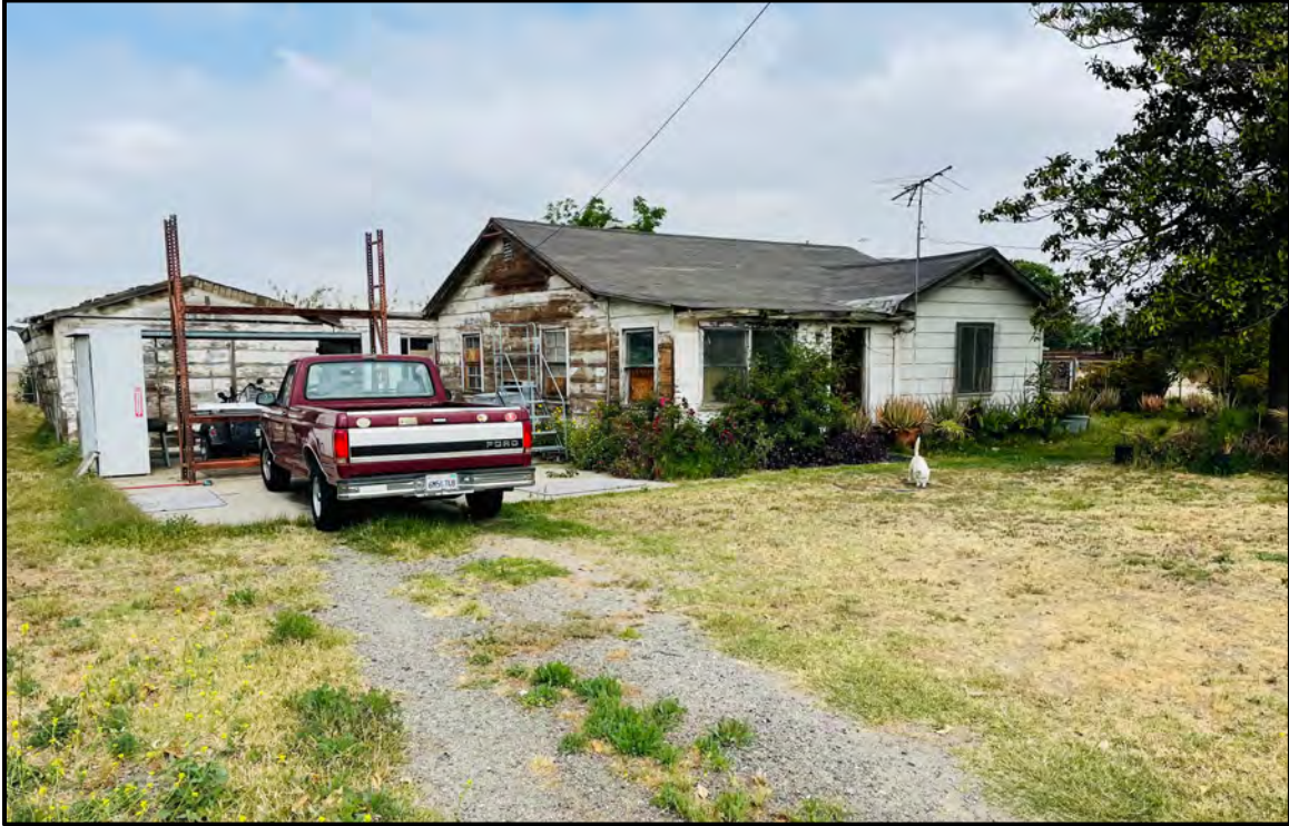
Plate 3.2–1: View of the residence and detached garage located at 10410 Locust Avenue, facing northwest.
