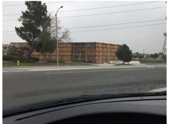
K-Rail Plywood & Acoustic Material
