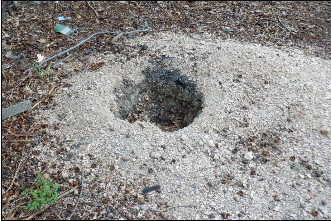
Figure 9. Soil Test Pit within Project Area.
