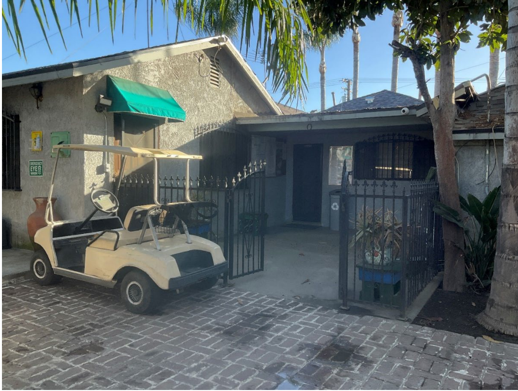
Figure 5-6. Northern elevation of building showing modifications for business use, facing east.
