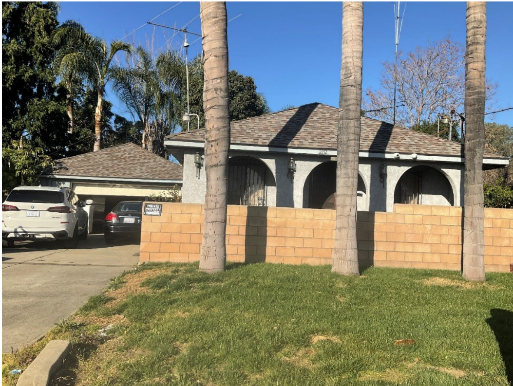
Figure 5-1. Overview of Project area from East End Avenue, facing west.
