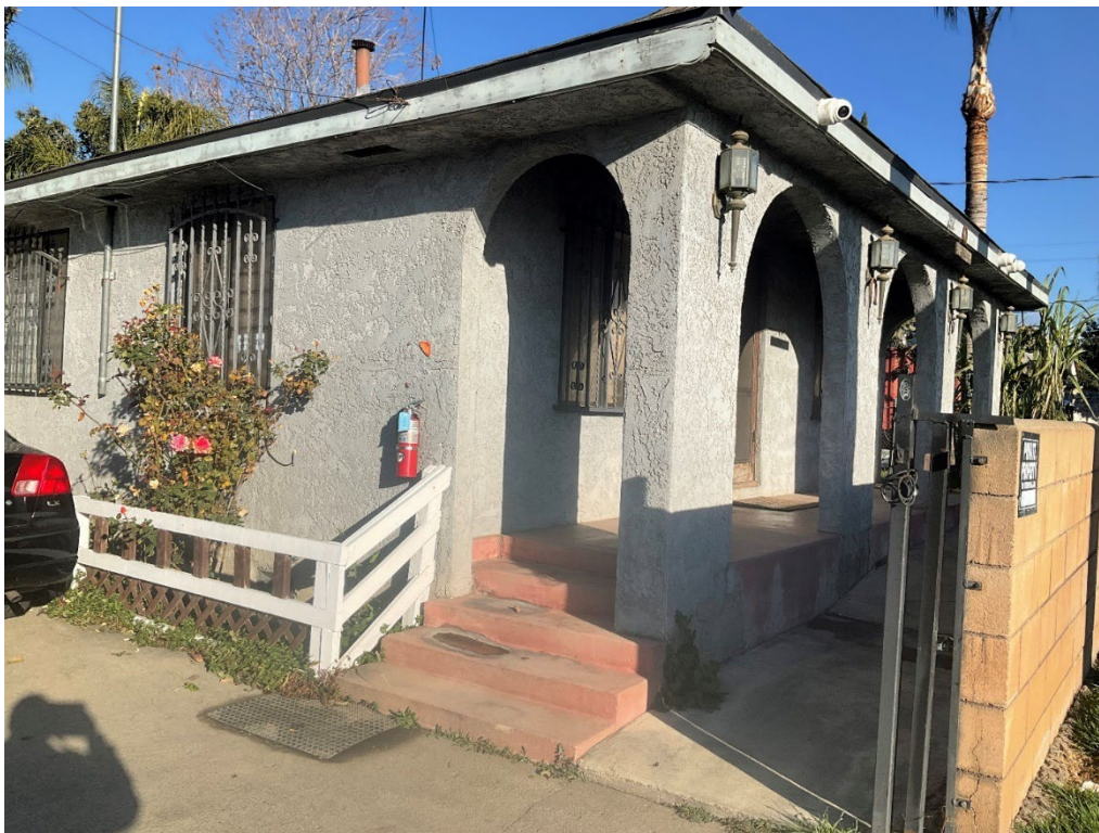
Figure 5-5. Eastern elevation of the building, facing northwest.
