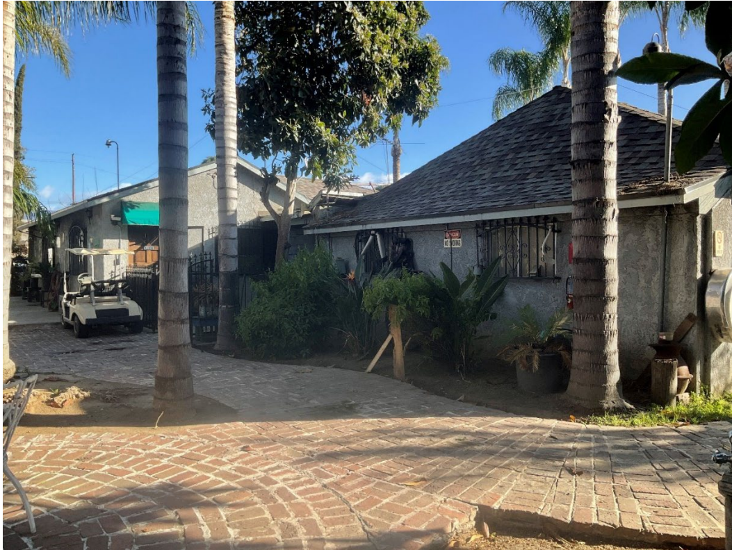
Figure-5-3. View of landscaping plants and ground coverage around the building, facing southeast.
