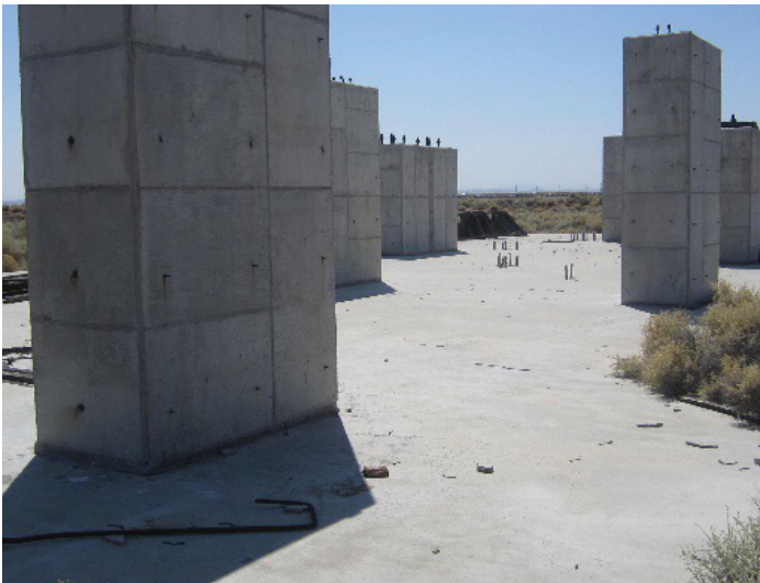
View of existing on-site SEGs X structure foundations.
