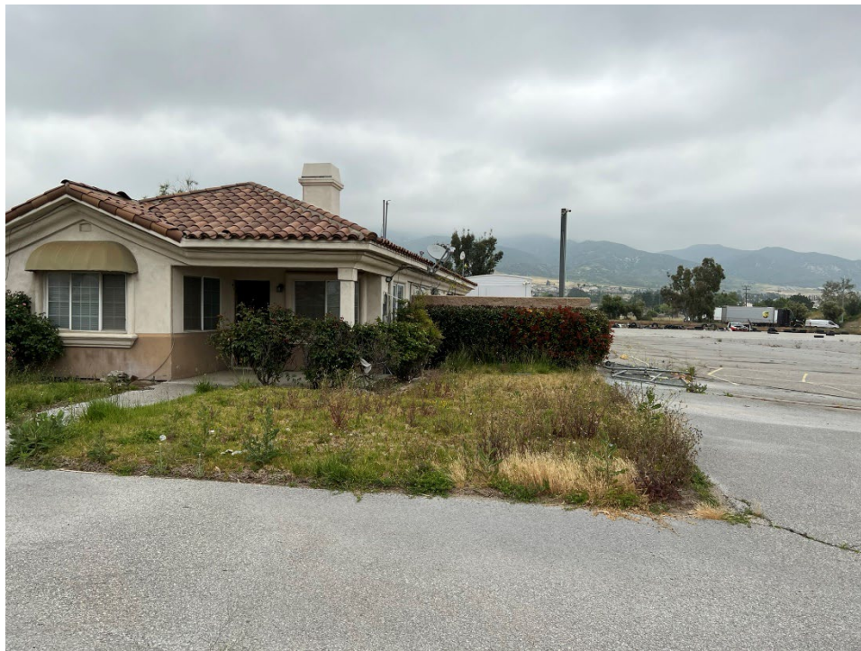
Photo 4 – Southwest boundary of the Project site, facing northeast.
