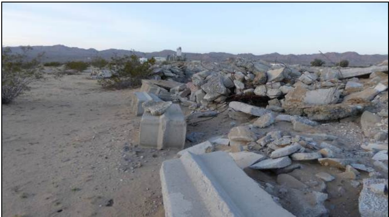
Photograph 10: Berm next to cement factory, facing South.
