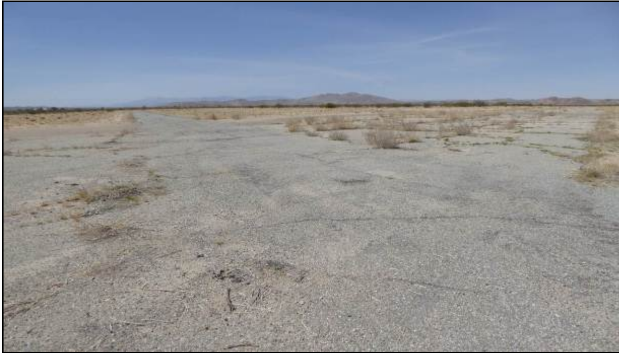
Photograph 13: Facing west from runway intersection. Note that annual burrweed and Russian thistle are beginning to grow in cracks in runway.
